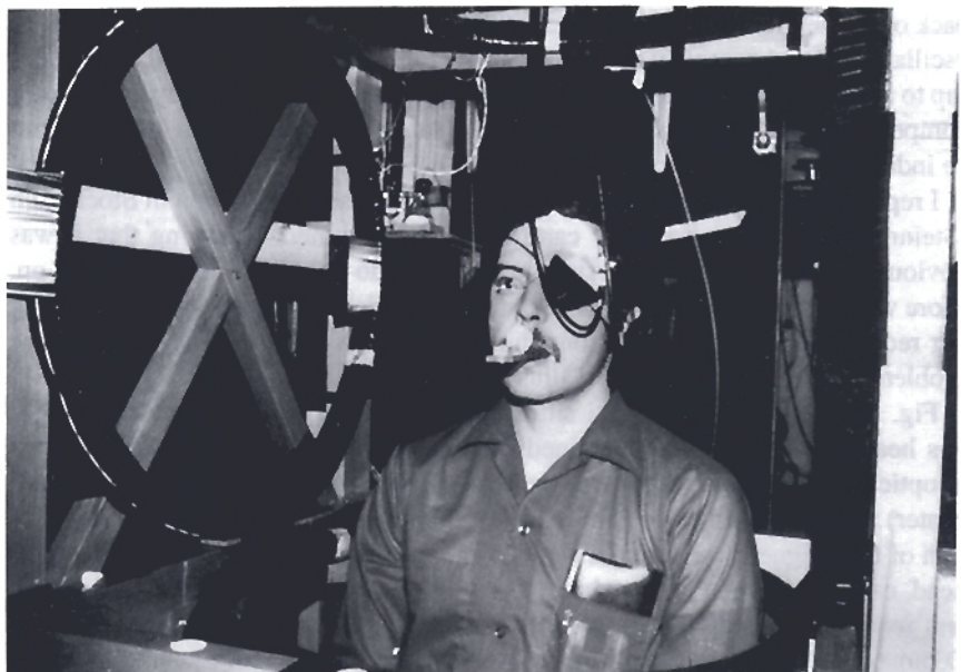
FIGURE 1.6. Alex Skavenski sitting in his magnetic field instrument having movements of his head and right eye measured by means of the amplitude-detecting technique (from Steinman, 1975).
