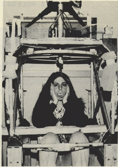
FIG. 13. Kowler in position for two-dimensional recording of rotations of her head by means of the magnetic-field search-coil technique. The head search coil is mounted on a dental bite plate. The field coils can be seen surrounding the subject who is using her hands to support her head.
